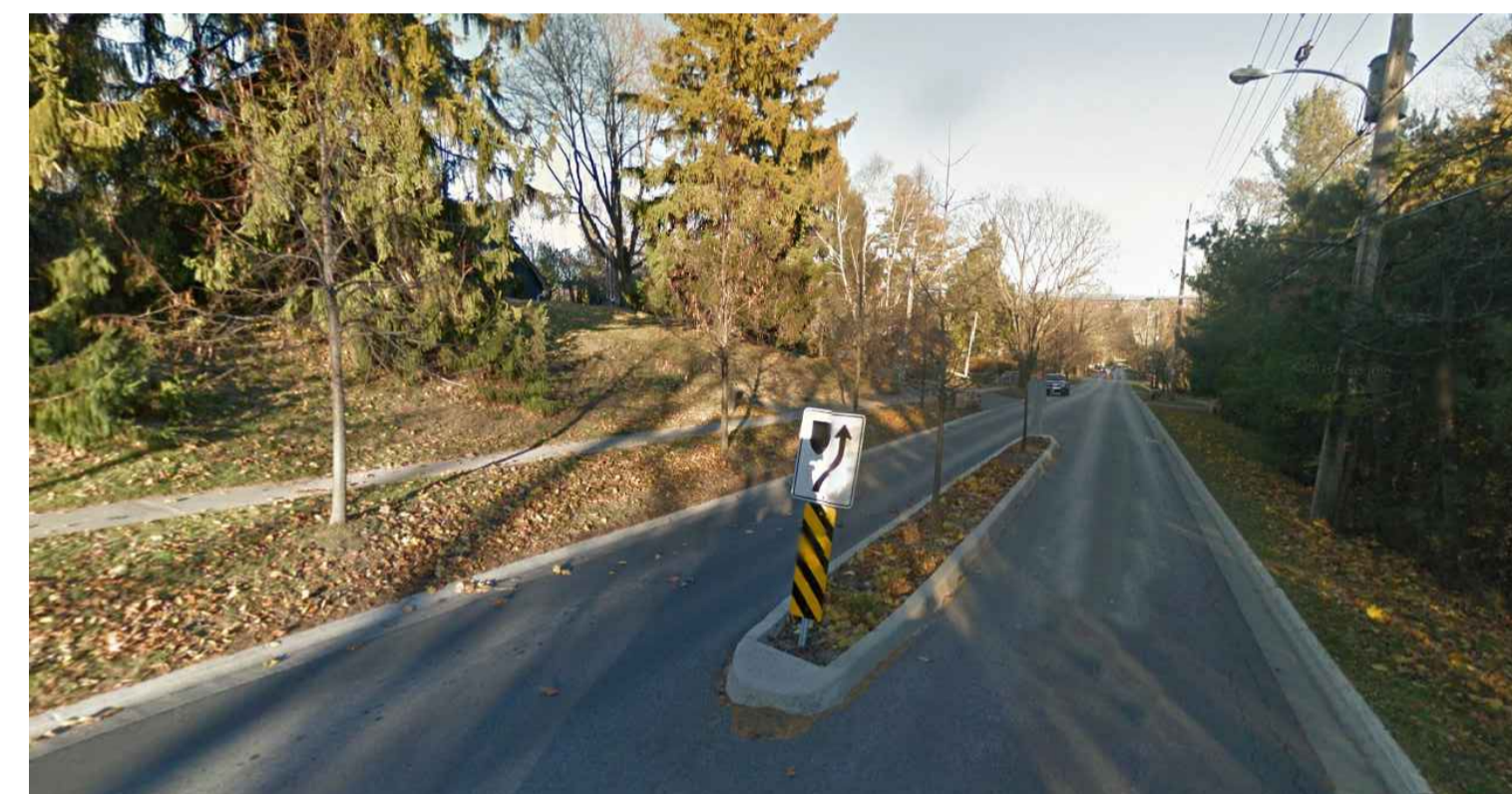
RAISED MEDIAN (Dorset Street, Port Hope, Ontario)
