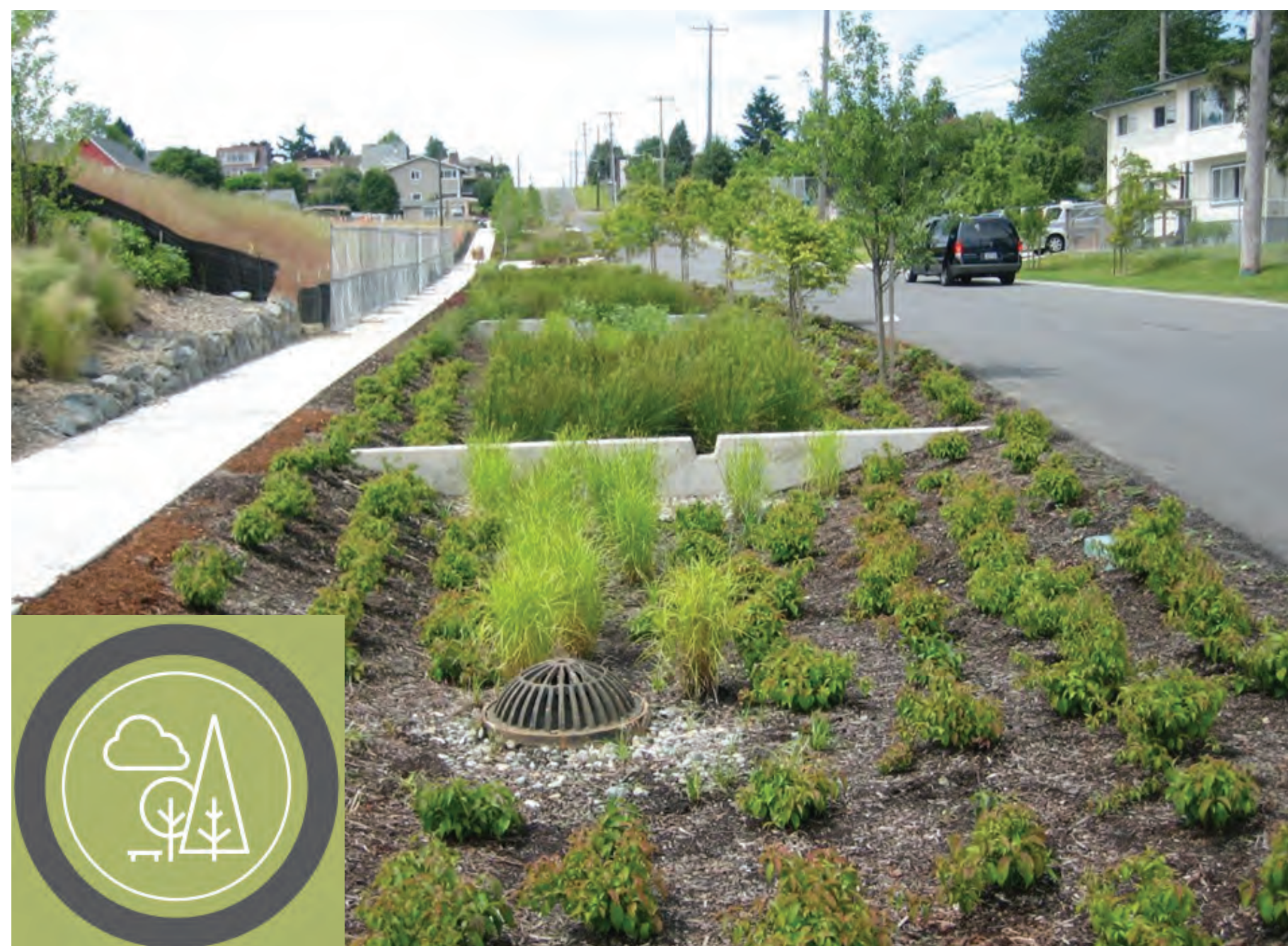
Green infrastructure which minimizes stormwater runoff and improves water quality - including bioswales, rain gardens, green roofs and permeable pavers.
