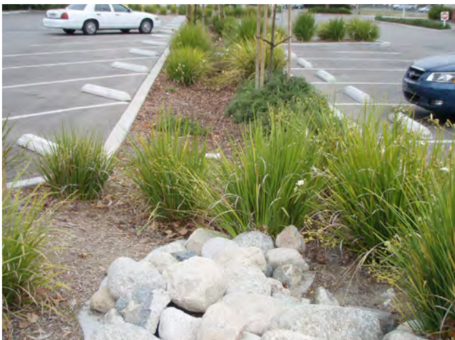
Landscaped island with a bioswale to filter run-off.
