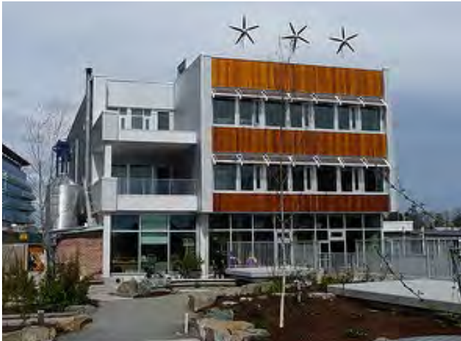
Wind turbines on the roof of an office building.
