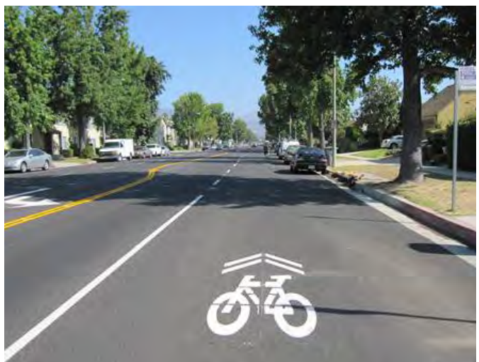
Clearly marked cycling lanes.
