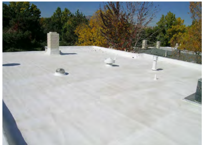
Light coloured roofs have a high solar reflectance, which reduces energy cost and reduces urban heat island effect.
