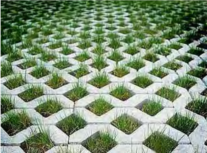
Permeable pavers to support on-site stormwater infiltration.
