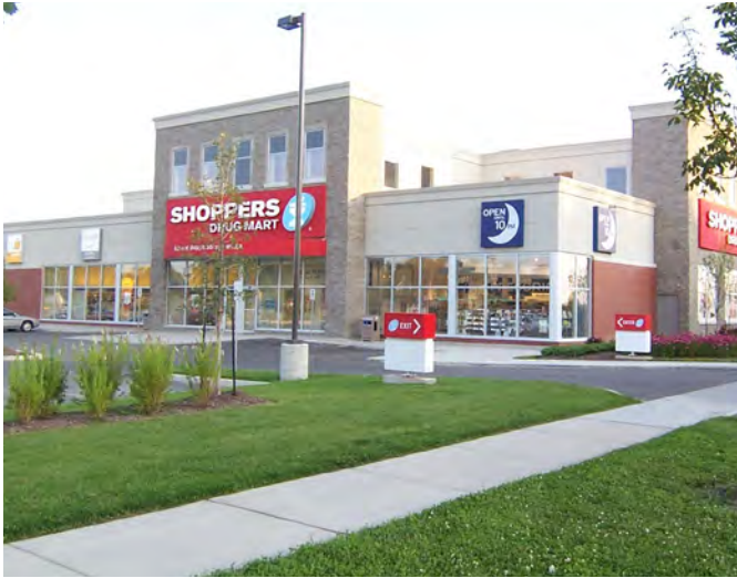
Example of a commercial building.
