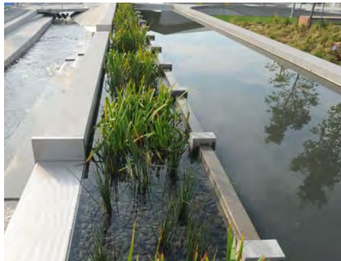
Innovative stormwater management facility.
