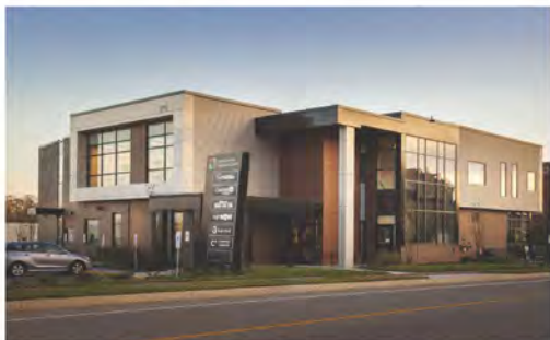
Small service offices (Medical Arts Centre, Guelph)
