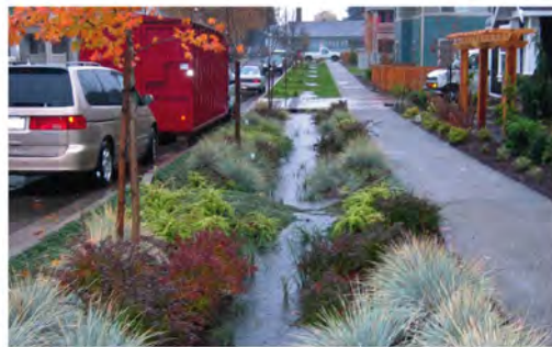
Low-impact development stormwater management
