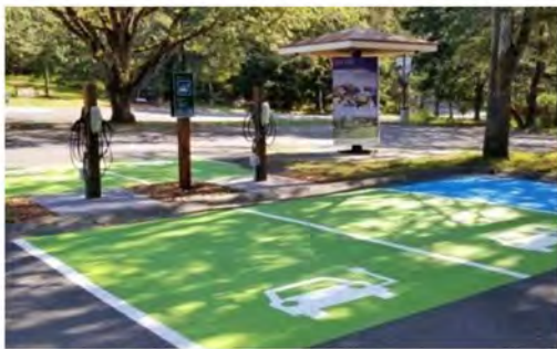
Electric vehicle charging stations
