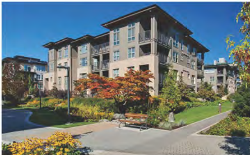
Low rise apartments (Wesbrook Village, Vancouver)
