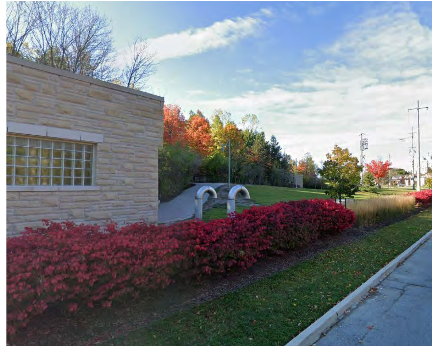
Landscape Treatment and Public Path at Ajax Watering Treatment Plant
