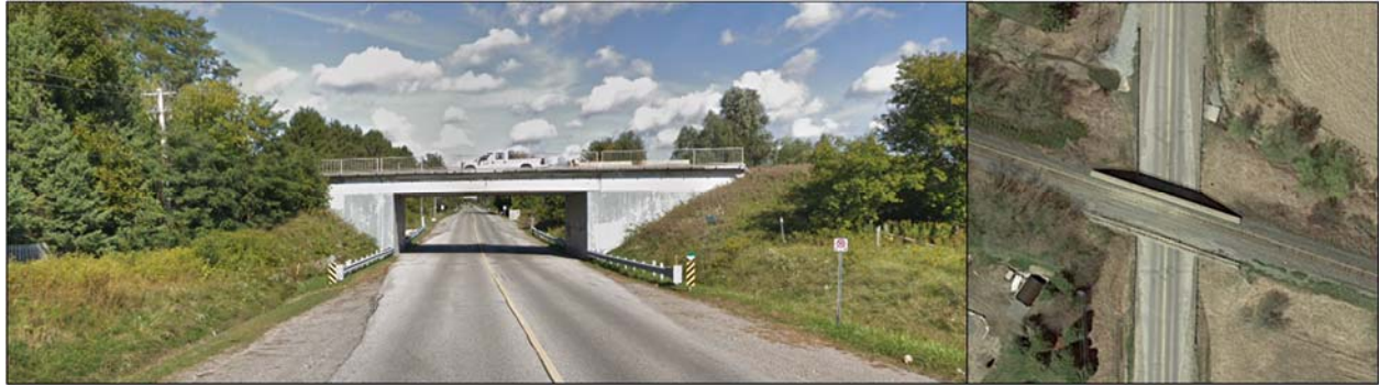
Figure 10: North Street & CP Rail Grade-Separated Crossing
