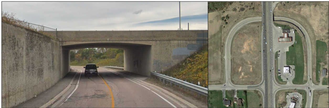
Figure 12: Concession Road 4 & Highway 34/115 Grade-Separated Crossing
