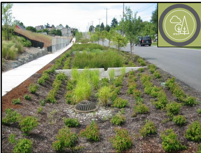
Green infrastructure which minimizes stormwater runoff and improves water quality - including bioswales, rain gardens, green roofs and permeable pavers.
