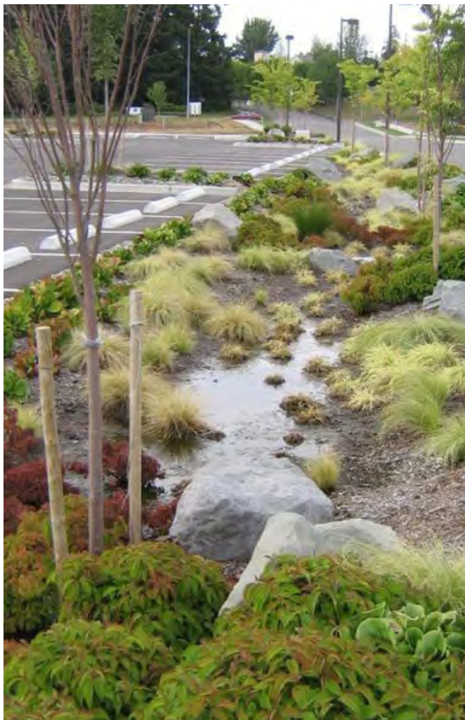
Figure 62: Example of Bio-retention Area
