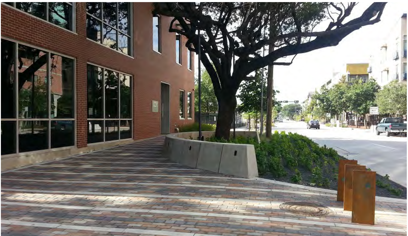
Figure 16: Example of Sidewalk
