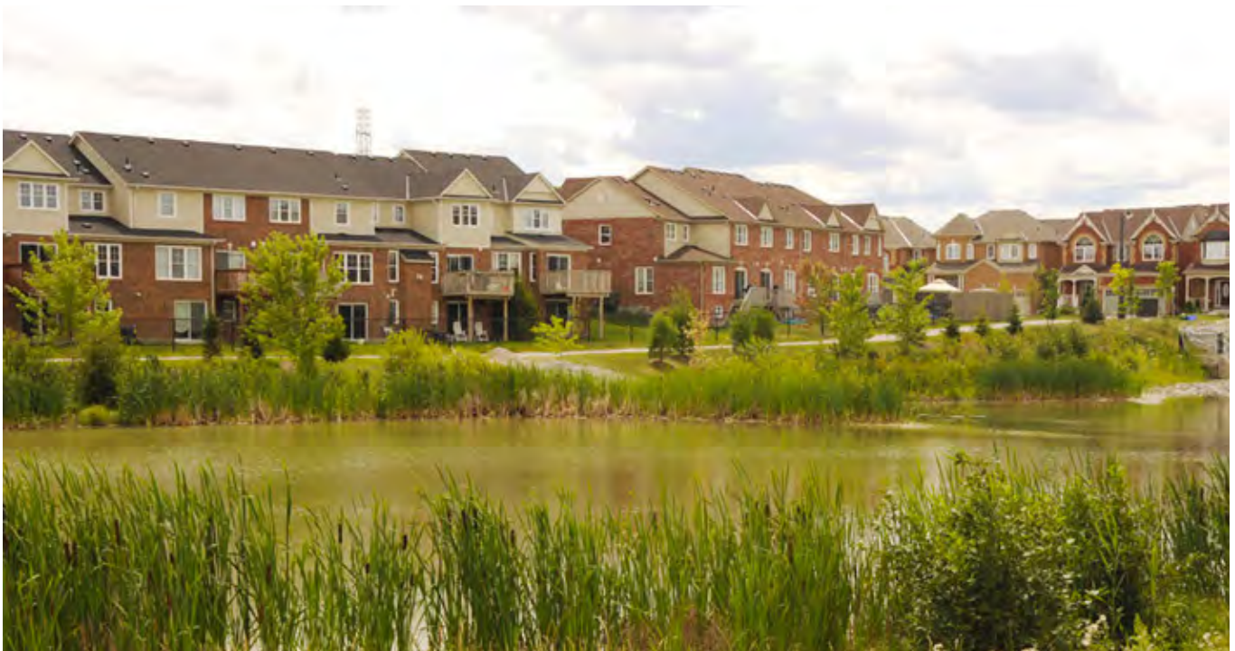
Figure 63: Example of Stormwater Management Pond
