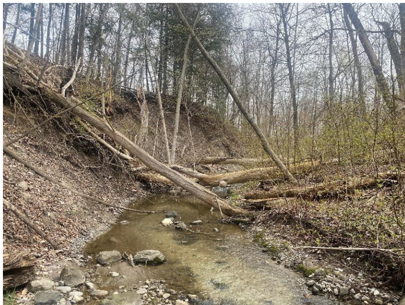
Photo 4. Looking downstream where Brookhill Tributary has locally eroded the toe of its valley wall.
