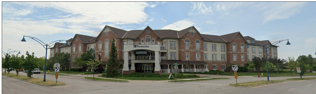
Figure 19 – Streetview (65 Clarington Blvd)
