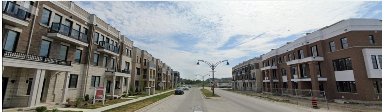
Figure 18 – Streetview (Clarington Blvd)
