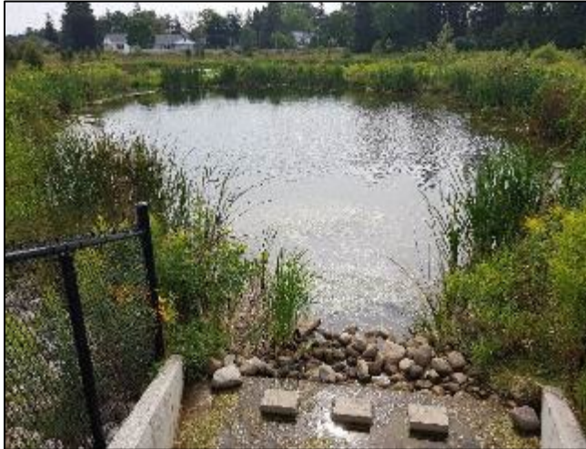
Figure 5.1: A wet pond SWM facility provides water quality treatment via the settlement of suspended pollutants and flood control via the temporary detention and peak flow reduction
