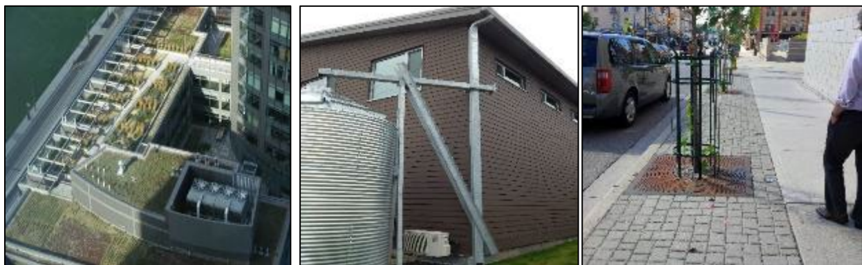
Figure 5.4: Example LID Practices from Left to Right: Green Roof (Portland, OR); Rainwater Harvesting (Portland OR); Permeable Pavements (London, ON)
