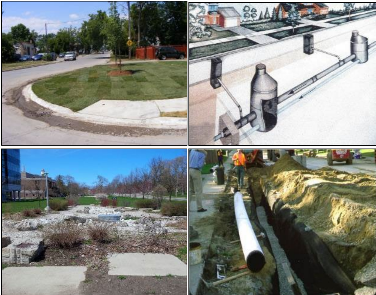
Figure 5.2: Example LID Practices from Top Left to Right: Soil Amendment (Mississauga, ON), Exfiltration System (Etobicoke ON); Exfiltration System (Guelph, ON); Perforated Pipe (Toronto, ON)
