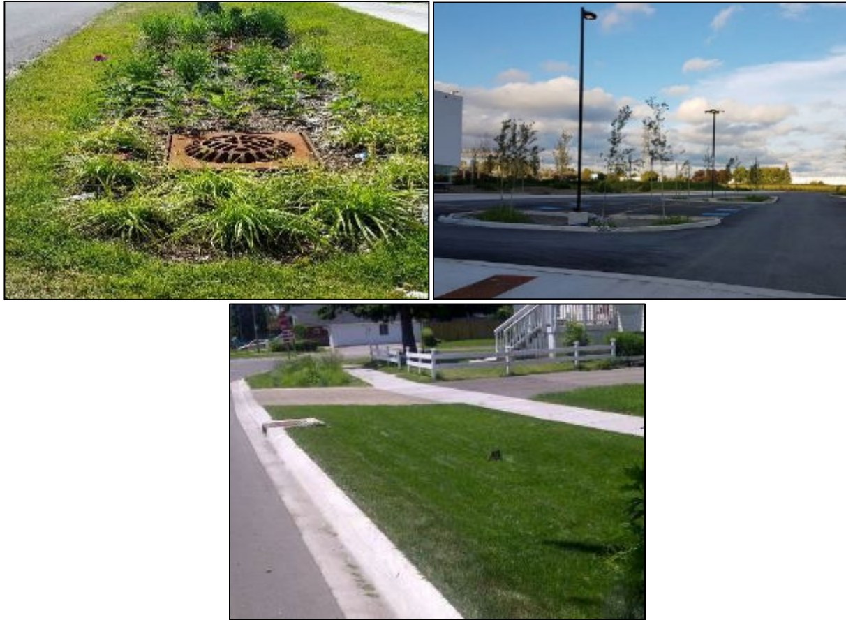
Figure 5.3: Example LID Practices from Top Left to Right: Bioretention (Toronto, ON); Bioretention (Bostwick Community Centre, London, ON); Grass Swale (Mississauga, ON)
