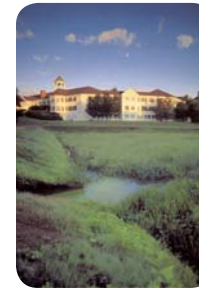
Storm water courses and ponds, together with the existing woodlots and hedgerows, should form the basis of a robust and attractive open space system.
