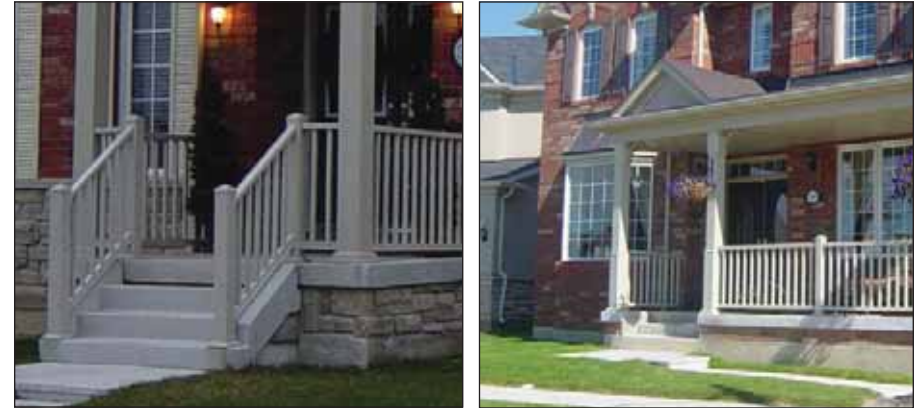
STAIRS SHOULD BE DESIGNED AS AN INTEGRAL COMPONENT OF THE DWELLING'S FACADE
