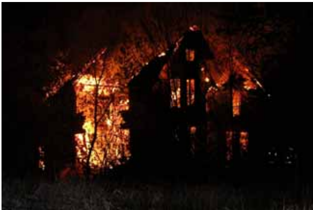
Structure Fire – Courtice
