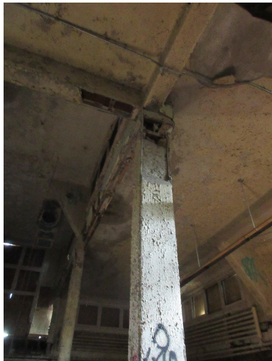
Photo 007 – Ground Floor Concrete Encased Beams and Columns
