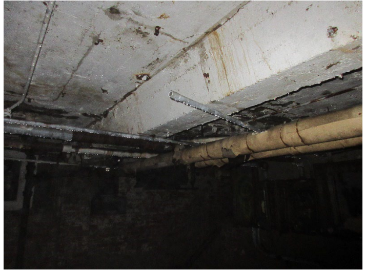
Photo 014 – Concrete Encased Beam
