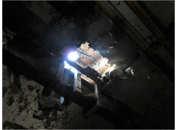
Photo 002 – Rotted Decking Viewed from below
