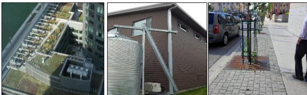
Figure 5.4: Example LID Practices from Left to Right: Green Roof (Portland, OR); Rainwater Harvesting (Portland OR); Permeable Pavements (London, ON)
