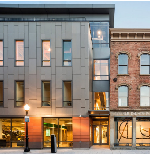
Figure 44: New development maintains a similar street wall height as the heritage building, with taller elements of the new development stepped back. The rhythm of punched windows with vertical orientation references the heritage facade. Where they join, the recess and high quality but contrasting materials does not compete with the heritage building, and allows each to contribute to a high quality street frontage.
