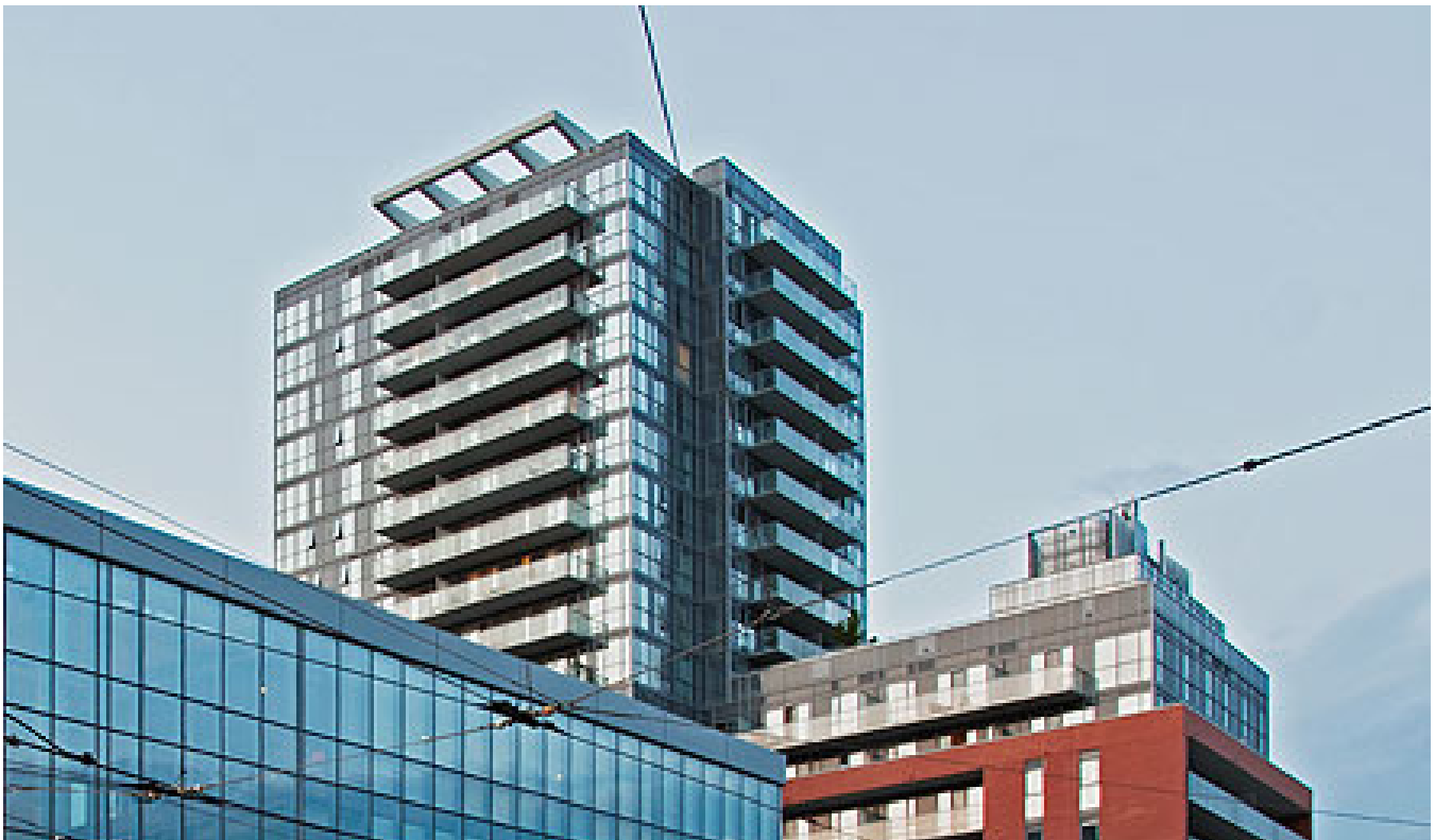
Figure 19: Mechanical penthouses set back from the edge of the building have an architectural expression different from, but consistent with, the facade, while contributing to an interesting skyline.
