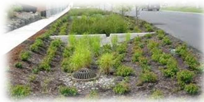
Implement Stormwater Management techniques that utilize natural drainage patterns to minimize the risk of flooding (refer to **Figure 39**).
