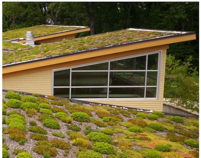
**Figure 7 :** Rain gardens, bioswales and green roofs are low impact development features that reduce runoff
