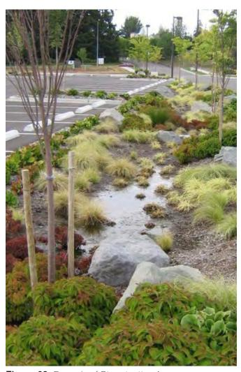
Figure 62: Example of Bio-retention Area
