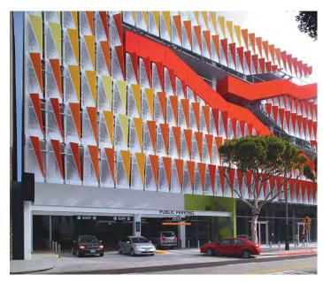
Figure 19: Example of Screened Structured Parking
