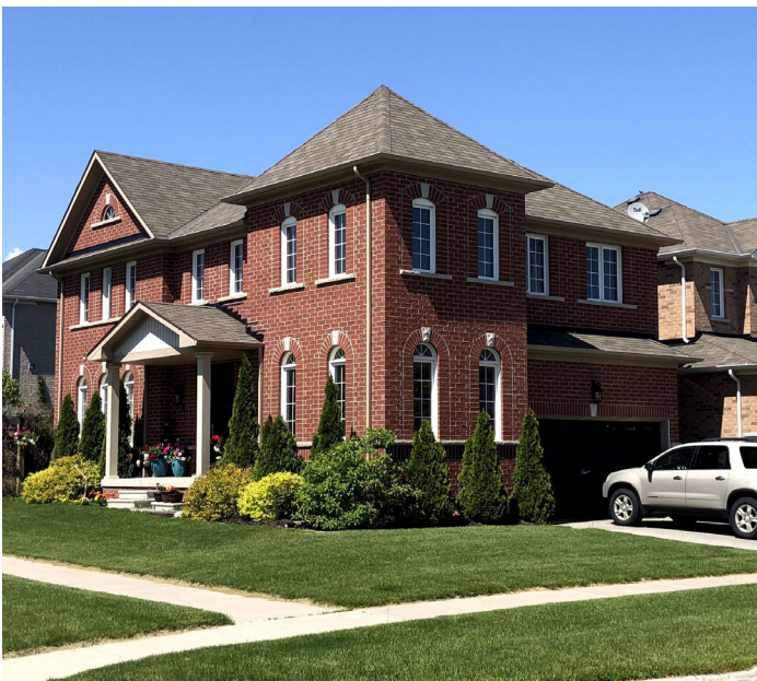
Corner lots should have built form and landscaping that appropriately addresses both streets
