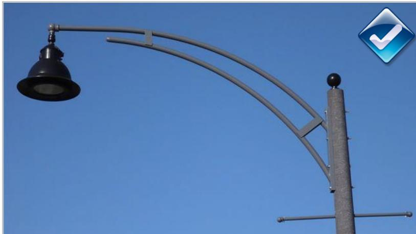
Figure 5: Full Cut-off Light Standard
