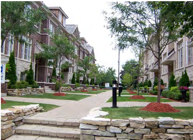
Townhouse units fronting onto a pedestrian walkway.
