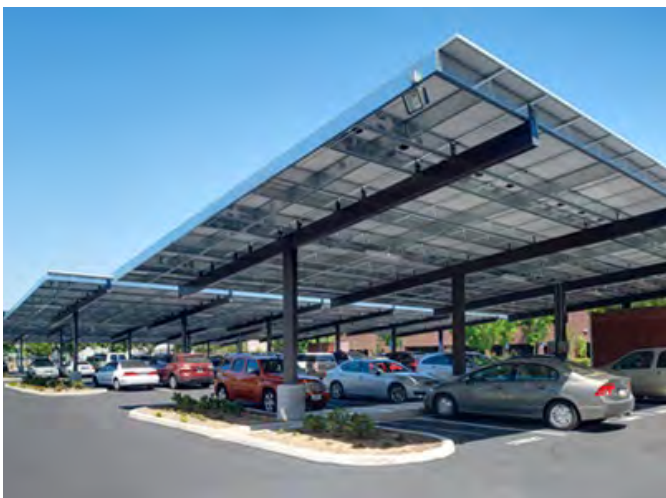
Solar canopies in surface parking lots.
