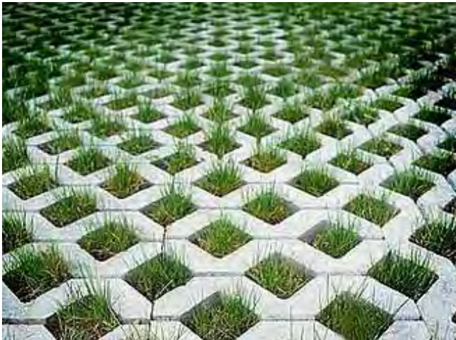
Permeable pavers to support on-site stormwater infiltration.
