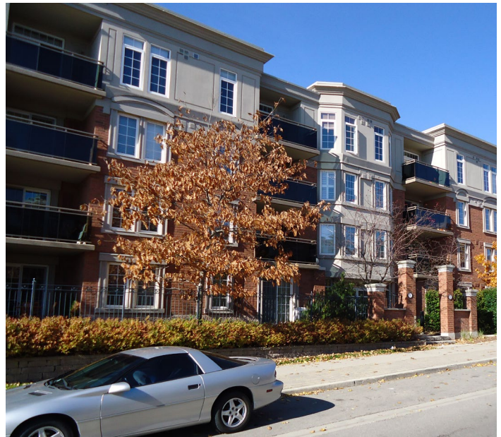
Low-rise apartment building with partially inset balconies and buffered patios
