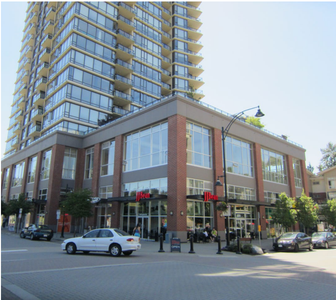
Tall building with a 2-storey podium and commercial uses on the ground floor
